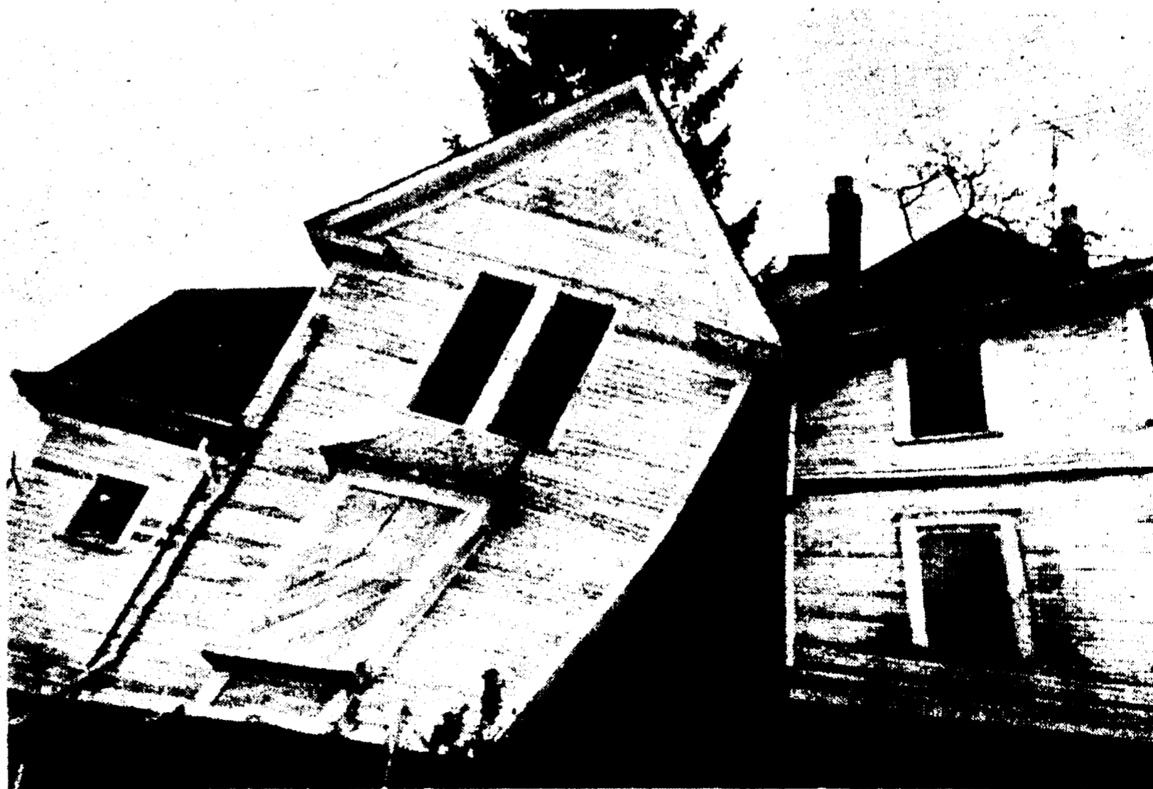
FOR A MOMENT Monday it was a lean - to, then this old two - story house on Main St. next to the Youth Center was demolished completely by a wrecking crew. (Staff photo by Hank Meijer.)
