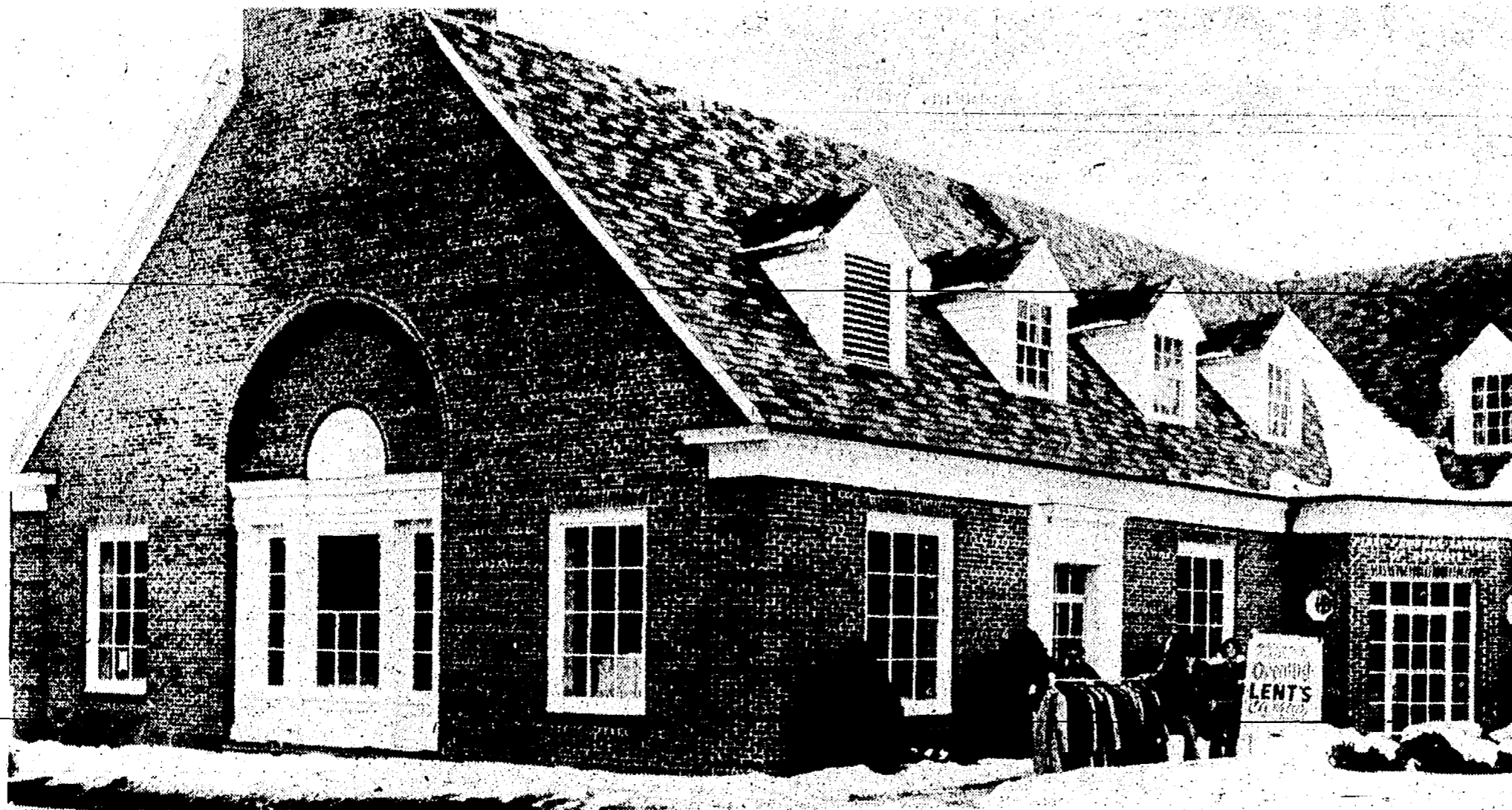
( Watch out for the carpenters! They're still working)
