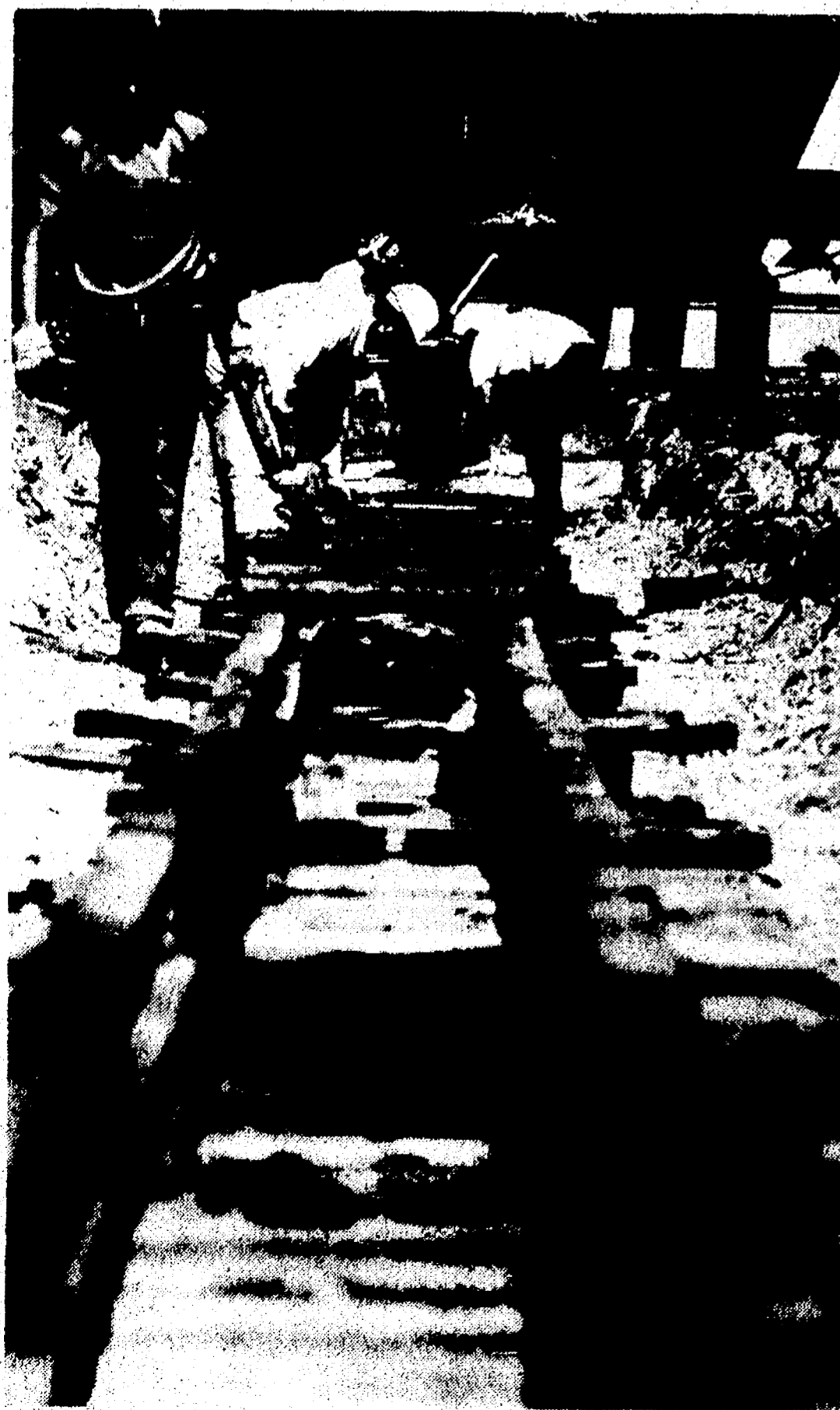
ROLLERS SPACED ALONG the track at even intervals carried the great tower forward.
