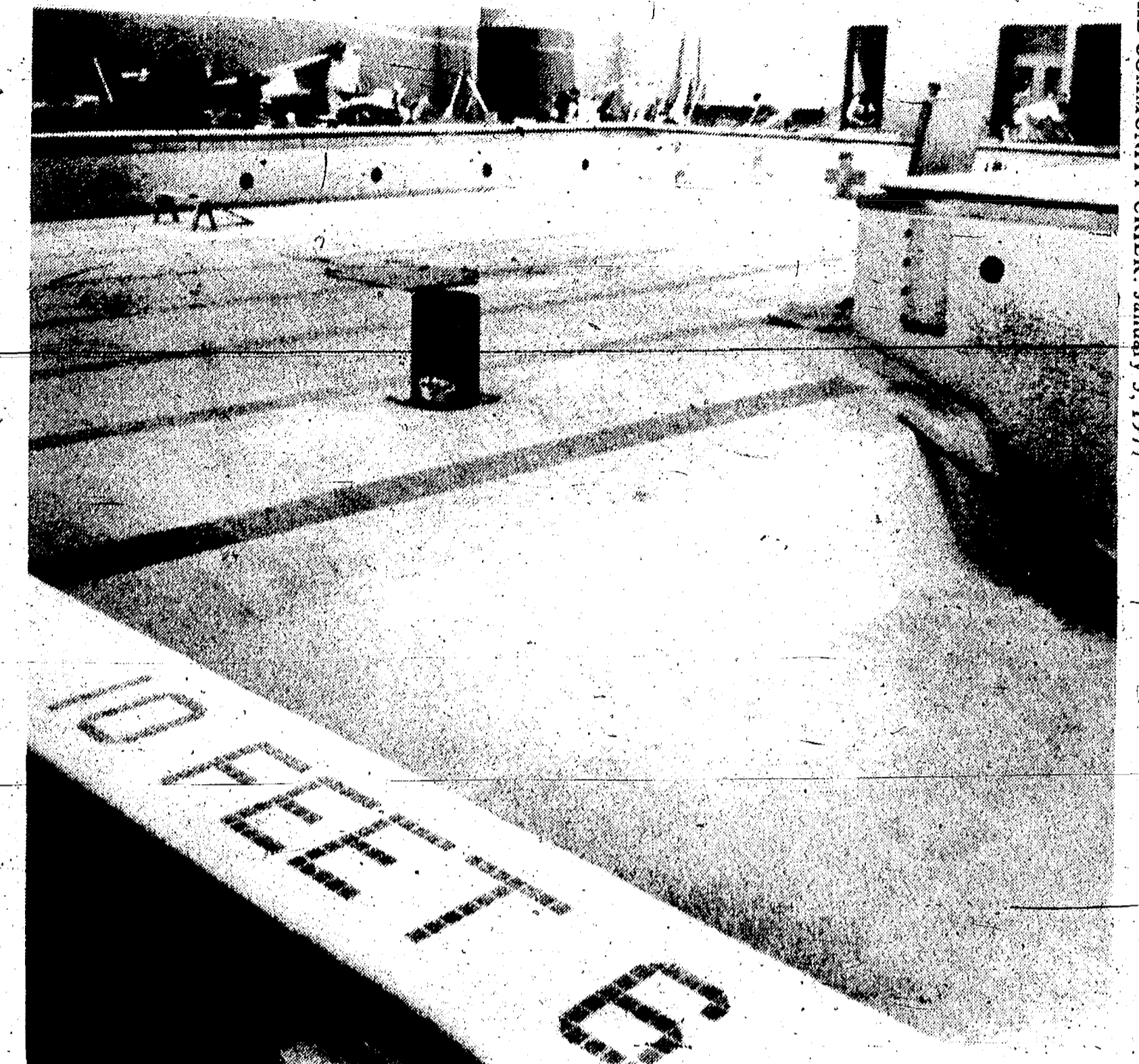
LAYING TERRAZZO TILE AROUND the new Phase III pool is a final step in the completion of the new physical education portion of the facility. The pool is of the same
