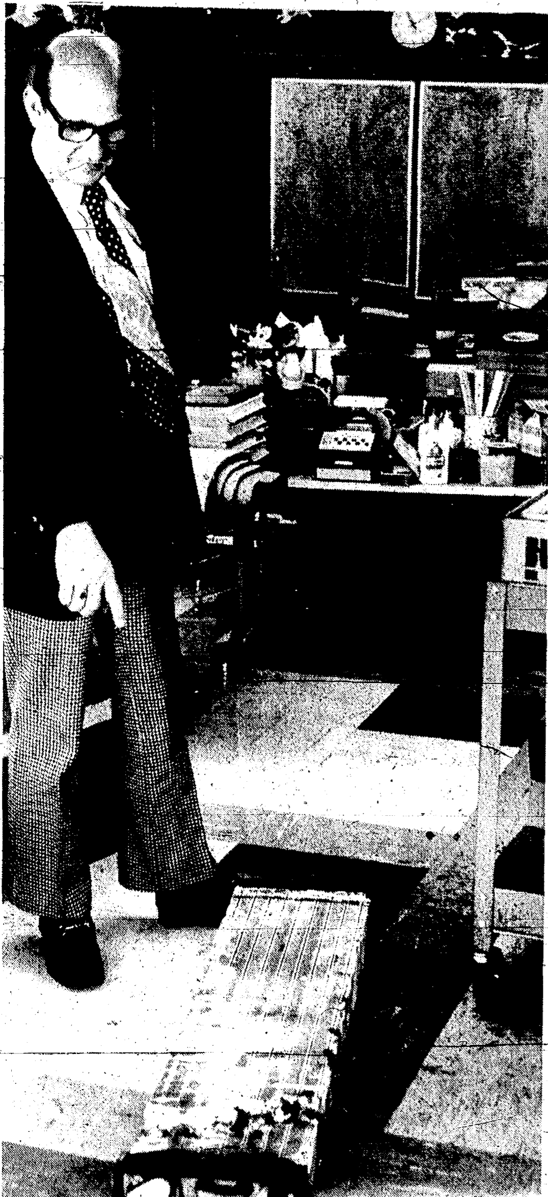
BROKEN HOT WATER PIPES at Farrand School over the weekend caused some flooding and heat loss at the school. Principal Earl Gibson examines the pipes which were replaced by workers early this week. (Crier photo by Hank Meijer)
