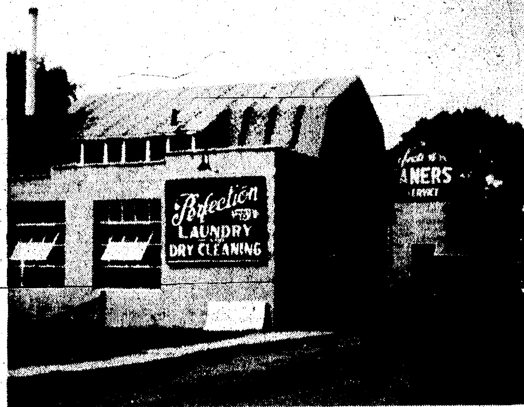
THE OLD PERFECTION LAUNDRY on Wing Street was remodeled from two cement block buildings and a frame house. The new building also added a second story. Several small shops replaced the laundry. These photos belong to the building's owner, Corey, and were submitted by Greg Green of Green's Glass, which occupies the east end of the building.
