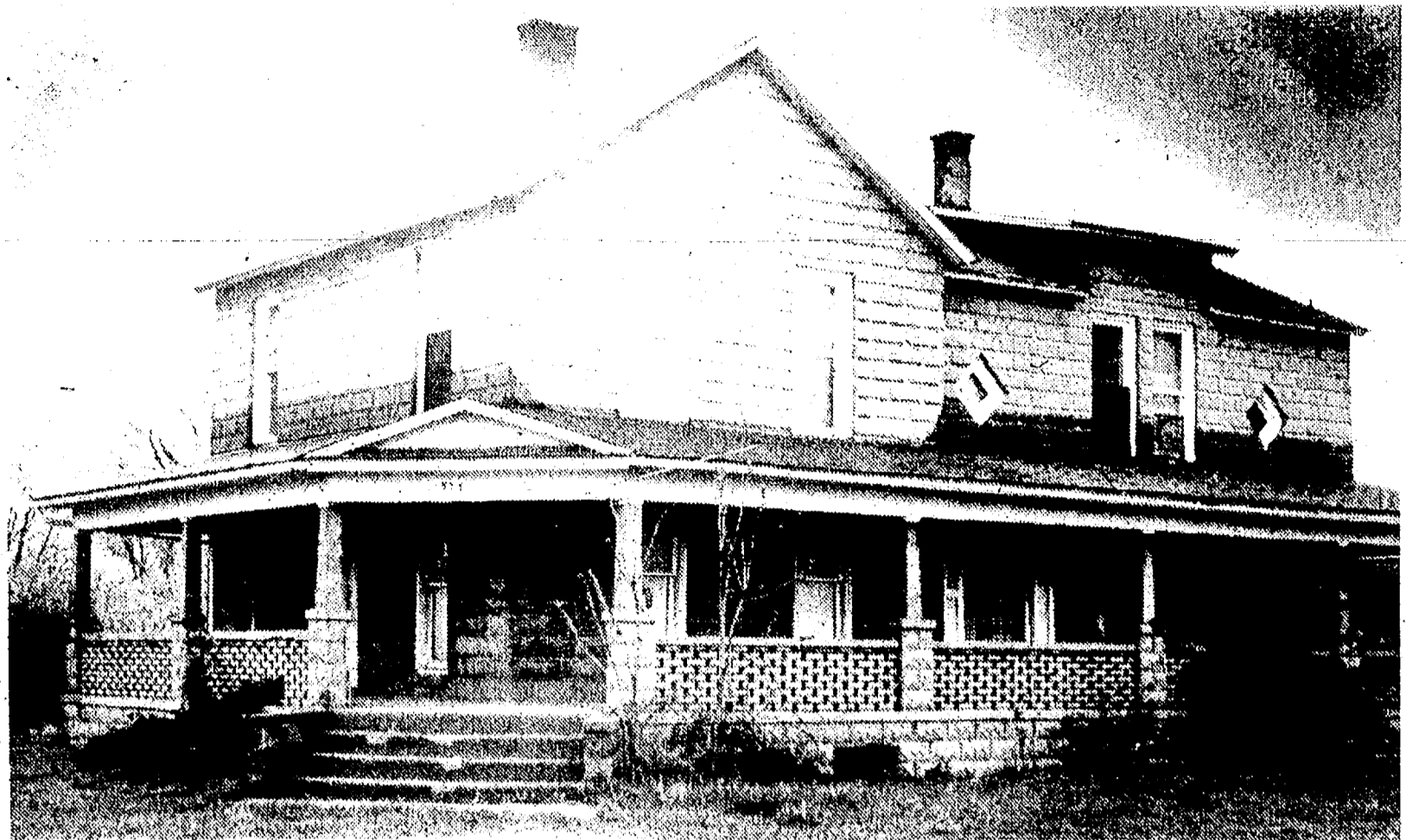
LEILA'S HOUSE stands condemned, waiting for the county to tear it down. front of our house for firewood."
