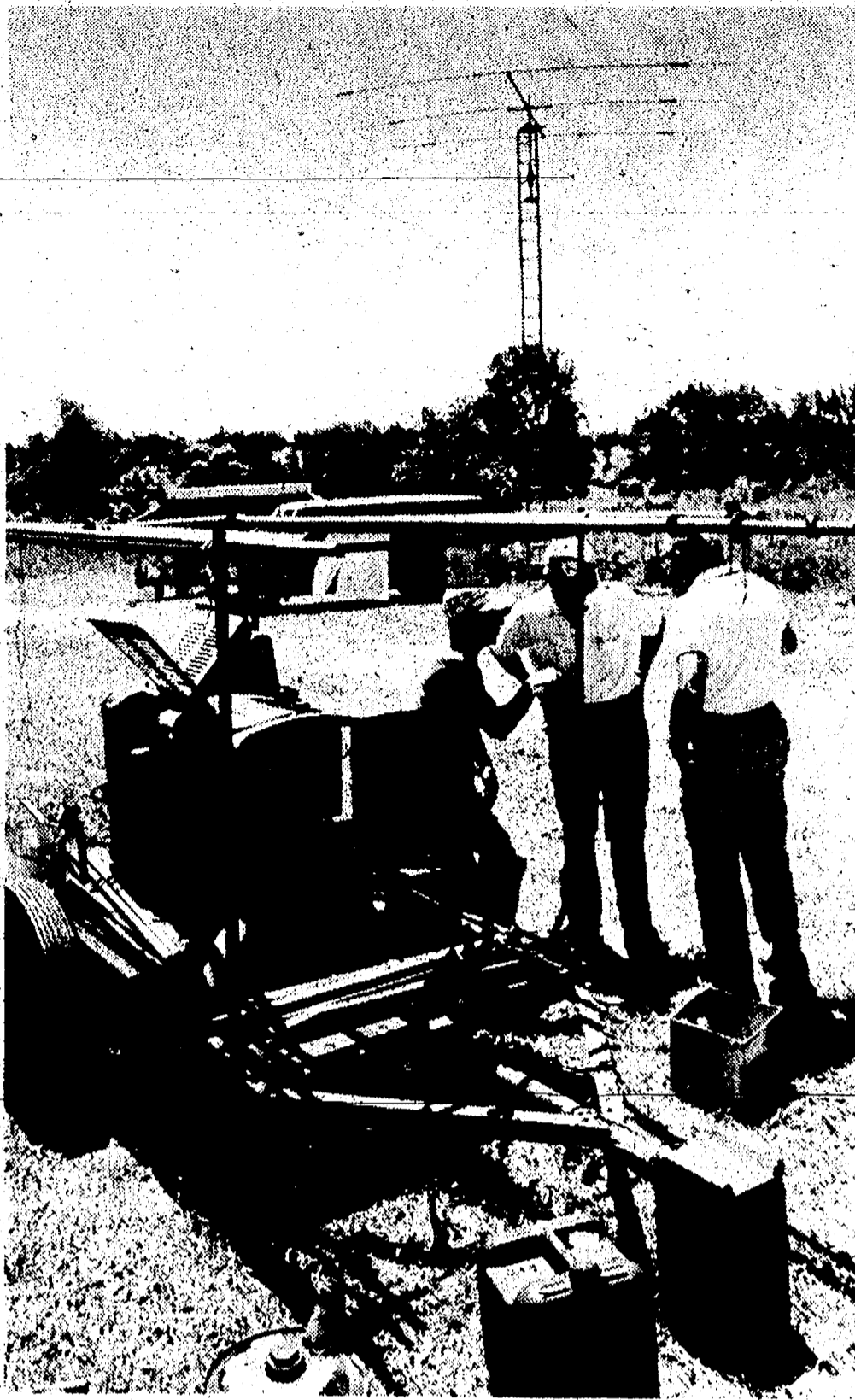
THIS PORTABLE GENERATOR provided power for 24-hours last weekend as members of the Plymouth American Radio Relay League made field contact with over 500 radio groups across the country.
