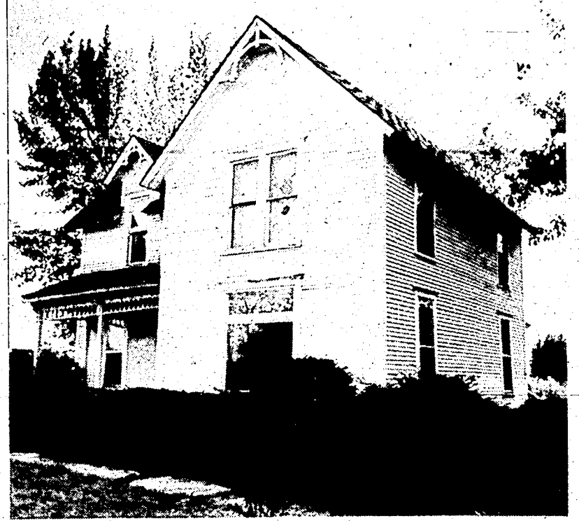
THE FOLKER HOUSE near Canton's new township hall on Proctor and Canton Center roads, will be restored and used as a social service center if the state approves grant money for the project. (Crier photo by Bill Bresler.)
