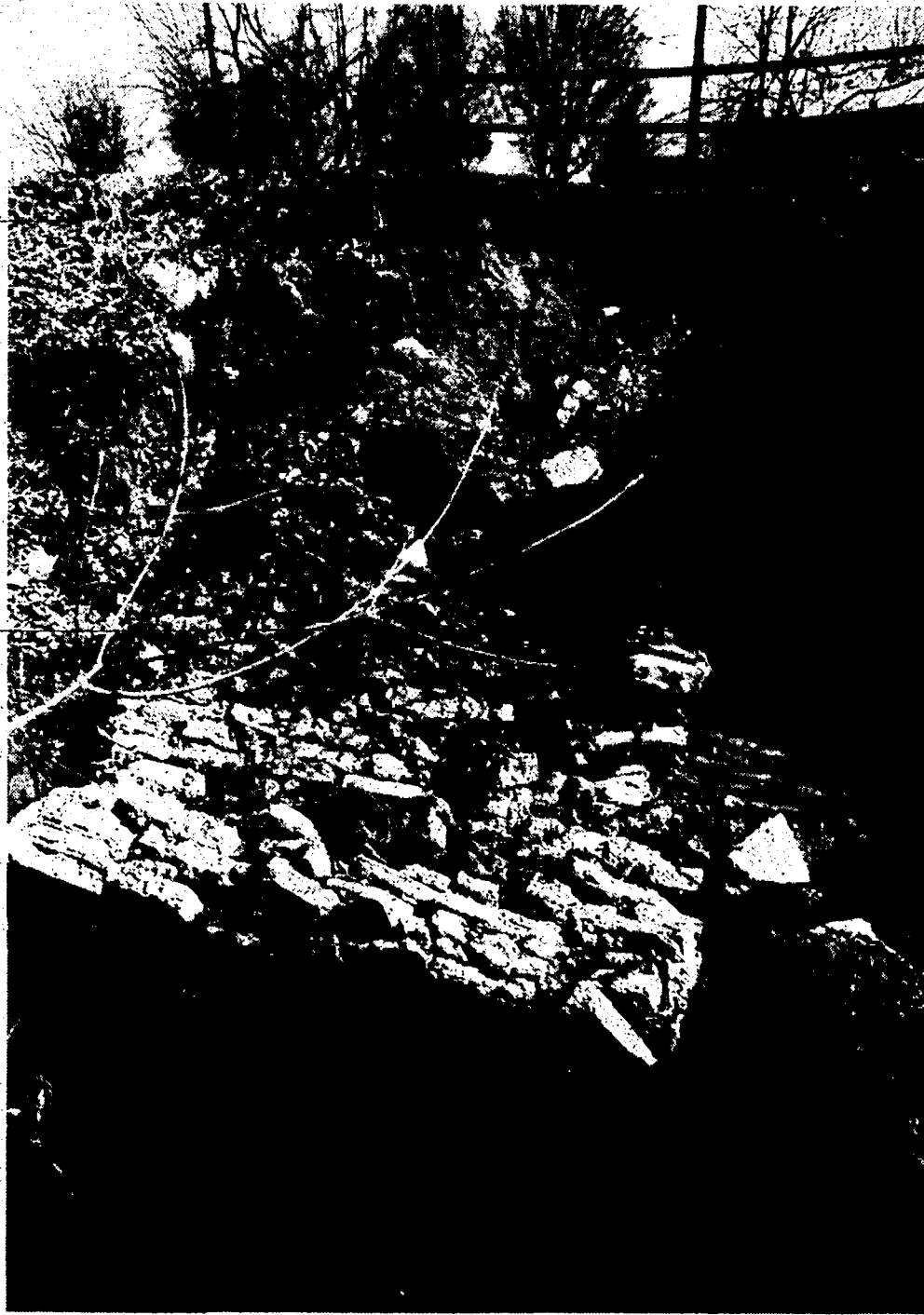
THIS CEMENT wall by the bridge at Coolidge and Burroughs streets has fallen, leaving a portion of the bridge unprotected against potential high water.
