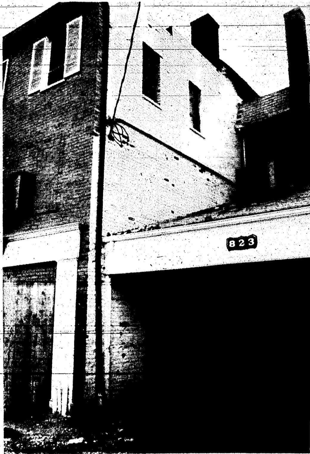
THE CITY of Plymouth may have to go to court to get this wall, the east side of the burned-out Penniman Avenue Shops, torn down. City Engineer Ken West believes it's a safety hazard, but a legal and insurance hassle is delaying its demolition. The wall is shared with the building of Morrison, Stanwood, and Polak, an accounting firm. Bricks from the wall are continuing to fall, said West. (Crier photo by Robert Cameron)
