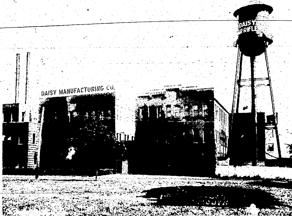
DURING the first half of this century, the backbone of Plymouth industry was the Daisy Manufacturing Co., makers of air rifles. In 1958, after 76 years in Plymouth, Daisy moved to Rogers, Ark. The plant now houses Adistra. This photo was taken in 1923. (Photo courtesy of Sam Hudson's "Pictures of Plymouth Past and Present")
