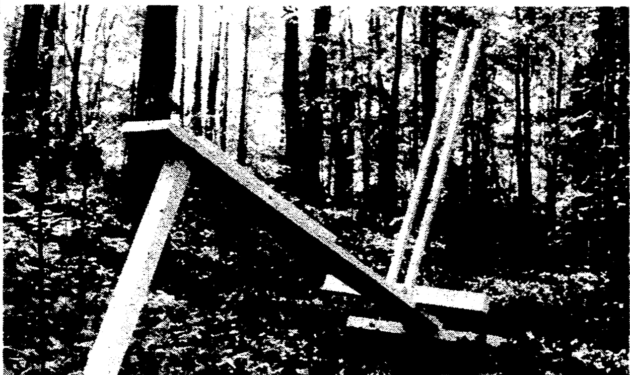
NEARLY COMPLETED is the Miller Woods Ski Jump, almost in time to host upcoming Olympic trials. The innovative structure, which does not rely on snow, is seen as the latest triumph of man over the elements.
