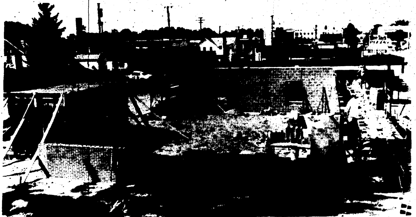
WORK IS PROGRESSING QUICKLY at the new branch of Down River Federal Savings and Loan
