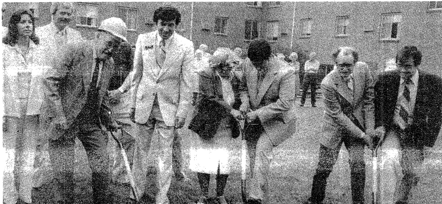
Tonquish Creek Manor celebrated their 25th anniversary in 1995. The senior housing complex has been an important part of the community ever since opening. This historic photo shows City officials at the ground breaking of the manor's addition.
