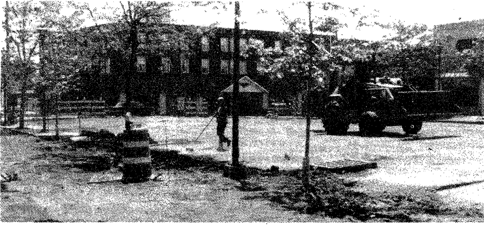
Plymouth Streetscape construction caused traffic headaches in 1995.
