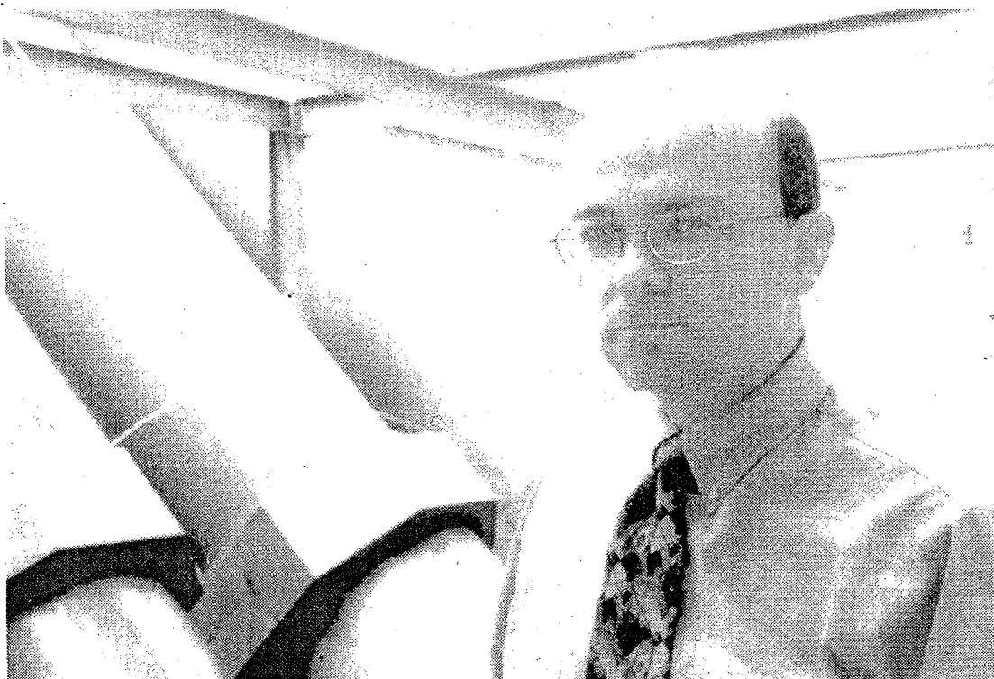
Canton's Tim Faas, operations manager of the Western Township Utility Association, has been on the job for a year and a half, making sure P-C-N's sewers are running smooth. The gigantic screw pumps behind him are capable of pumping 10,000,000 gallons of water a day to waste water treatment plants in Detroit and Ypsilanti. (Crier photo by Scott Spielman.)
