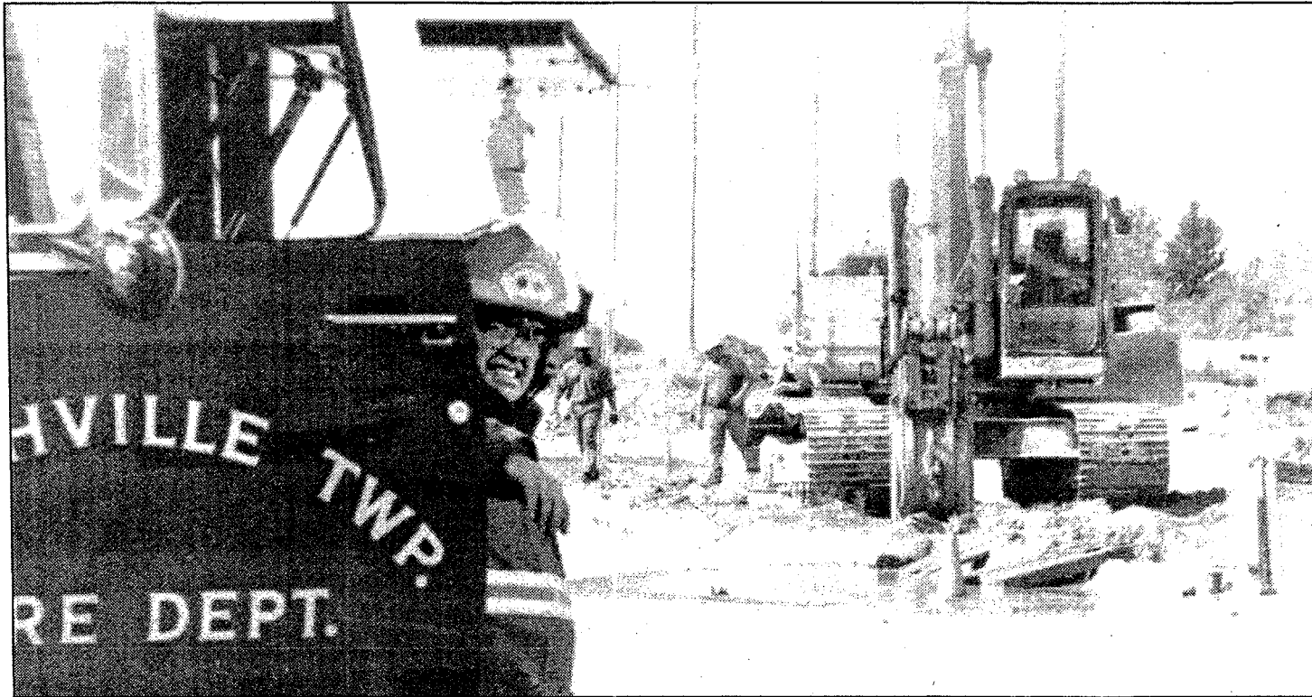
As firefighters from Northville Township and Plymouth look on, crews from Consumers Power repair a broken gas main at Beck and Five Mile roads Wednesday afternoon. Contractors hired by Detroit Edison struck the main with a backhoe (Crier photo by Scott Goodwin).
